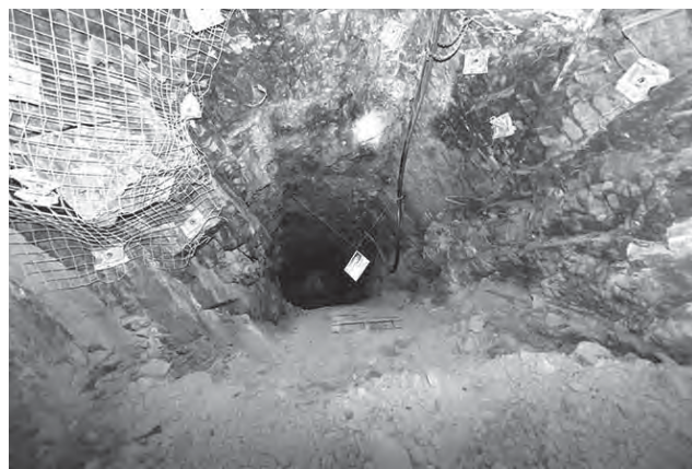
☆ Union Hill Mine: the sharp decline travelling underneath the township of Maldon.
